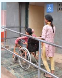
SPECIAL TOILETS FOR PEOPLE WITH DISABILITY
